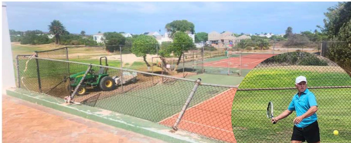
Caption: Repairs to the fence between the bowls club and Court 1 is underway.
